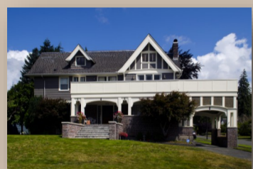
23 400 W 8th Street Built 1912 Tudor Revival
