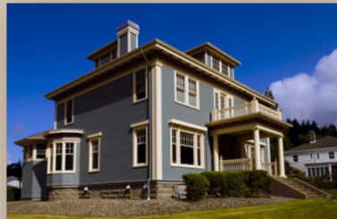
13 1005 N Broadway Built 1906 Federal Revival
